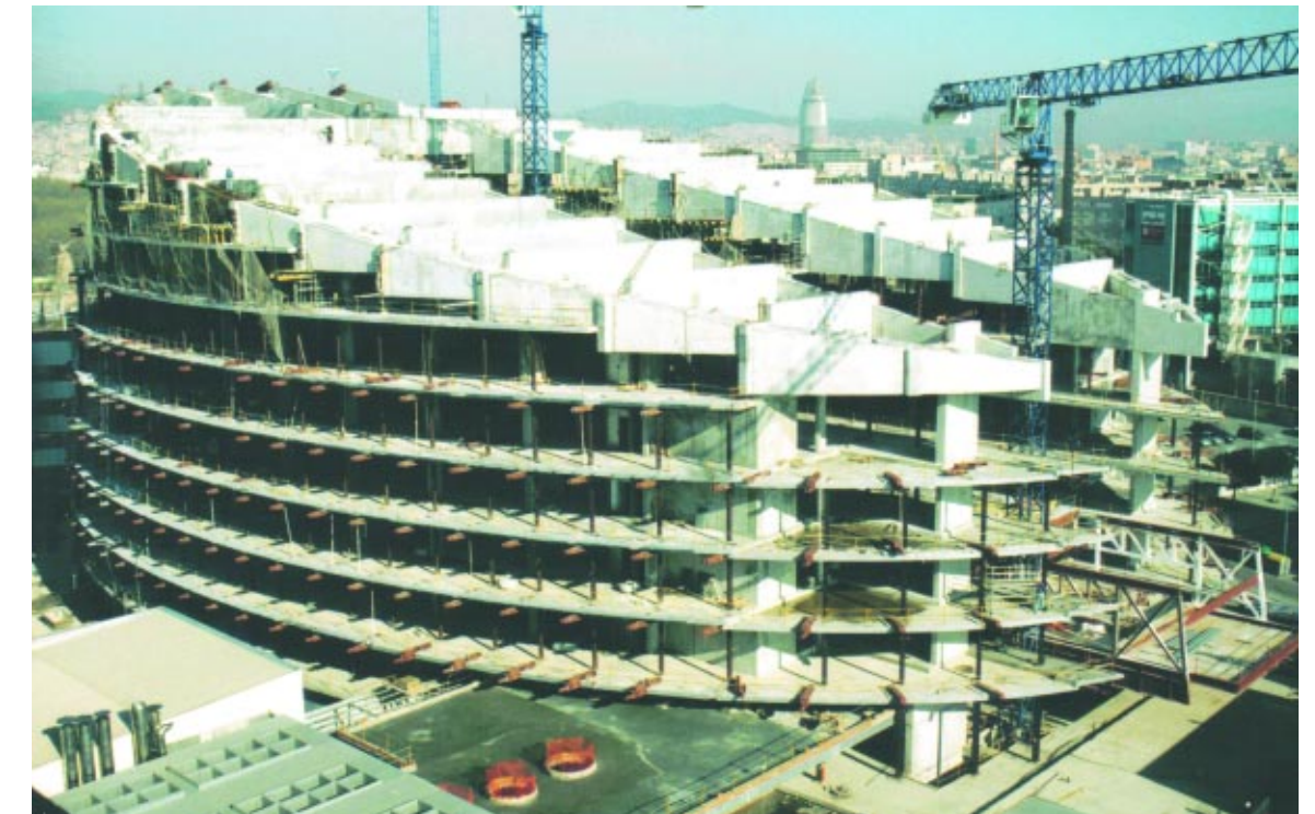
17. View of the upper suspension structure: main beams, internal strut and double external strut.
