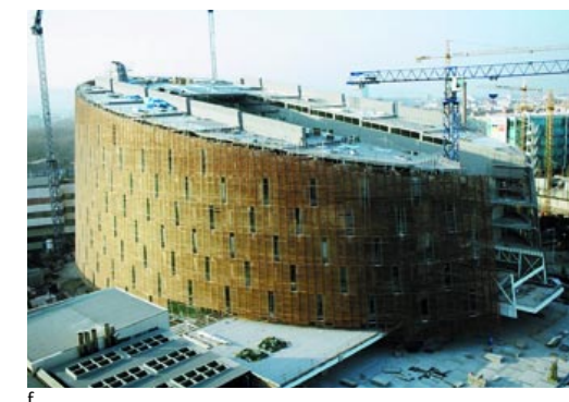
6. Sequence of the construction process. a. Constructing the propped decks (September 2003). b. Constructing the upper suspension structure (January 2004). c. Putting the upper suspension studs in place and anchoring the braces to the suspension structure (April 2004). d. Removing the props and suspending the building (September 2004). e. Constructing the exterior facade (December 2004). f. Completed exterior facade (March 2005).
