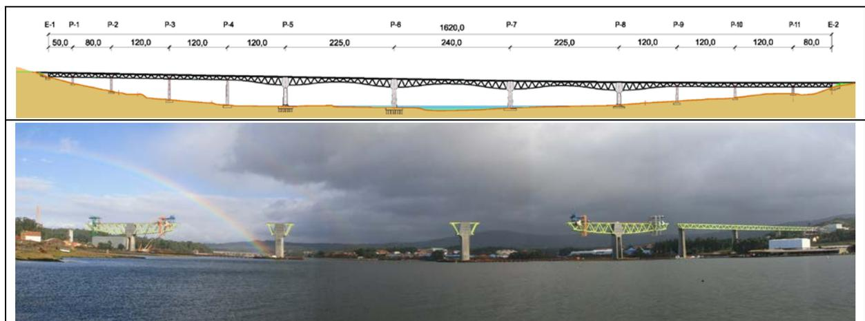
*Fig. 1.* a) Elevation view of the viaduct over river Ulla; b) Current state of the works (January 2014)
