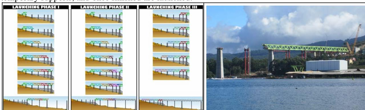
Fig. 6. a) Scheme of the constructive procedure by launching in three phases; b) View of the launching phase II.
