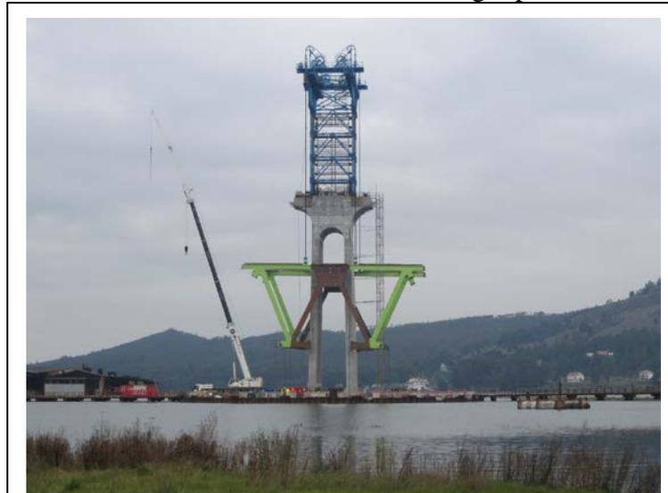
*Fig. 3.* View of the erection of the zero "W" steel segment over one of the central piers
