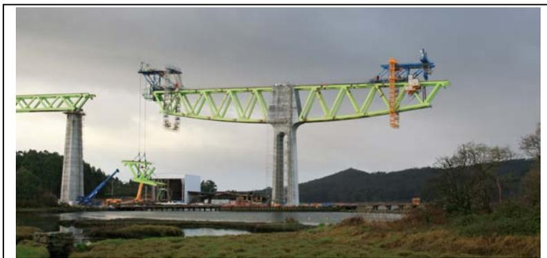
Fig. 5. View of the lifting of one segment of the main central spans, constructed by incremental equilibrated cantilevers
