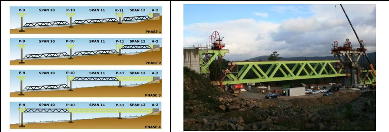
*Fig. 7.* Scheme of the constructive process of spans 10, 11 and 12; b) View of the lifting of span 12.
