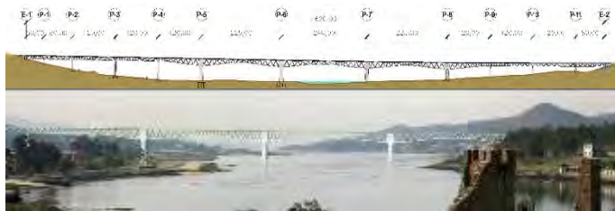
Figure 12. View of Viaduct over river Ulla
