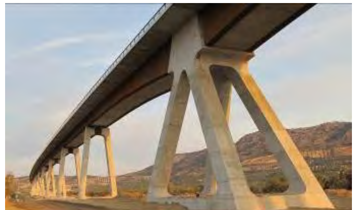
Figure 9. View of the central and typical piers of the Viaduct
