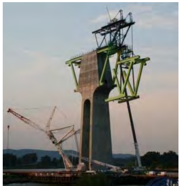
Figure 15. View of pier P-5 while erecting a segment
