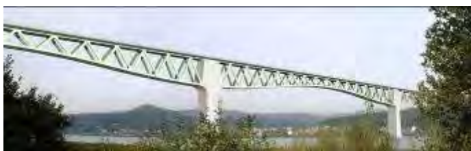
Figure 13. Lateral view of the main span of Viaduct over river Ulla
