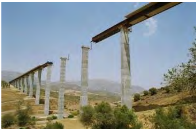
Figure 4. Underneath view during launching
