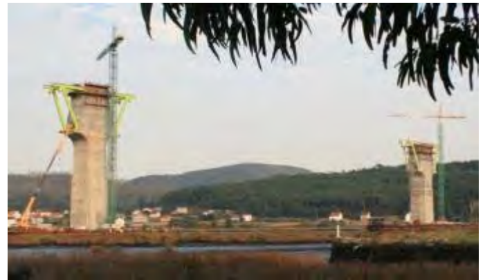
Figure 14. View of the two inner piers P-6&P-7
