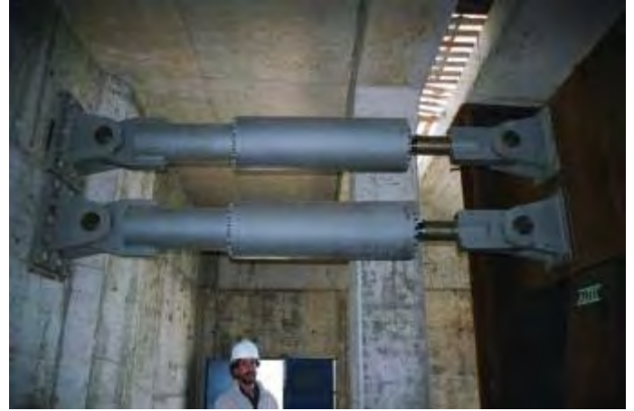
Figure 5. Longitudinal viscous damper-shock transmission
