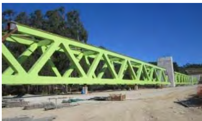
Figure 21. Approaching spans near abutment 2 (120+120+80 m) ready for vertical lifting.
