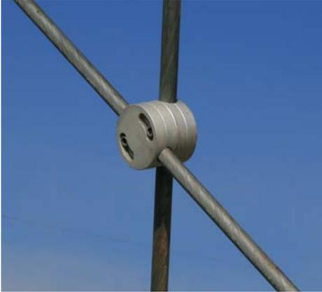
**Fig. 12:** Palma del Río's cable hanger crossing device
