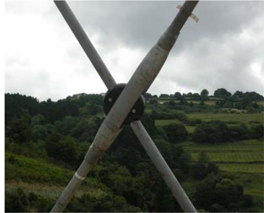
**Fig. 13:** Deba's rod hanger crossing device
