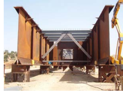
Fig 7: Steel twin girder system
