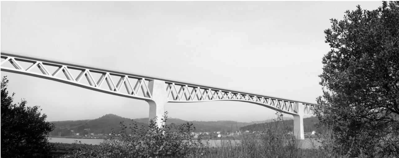
Fig. 4. Lateral view of the main span of Viaduct over river Ulla
