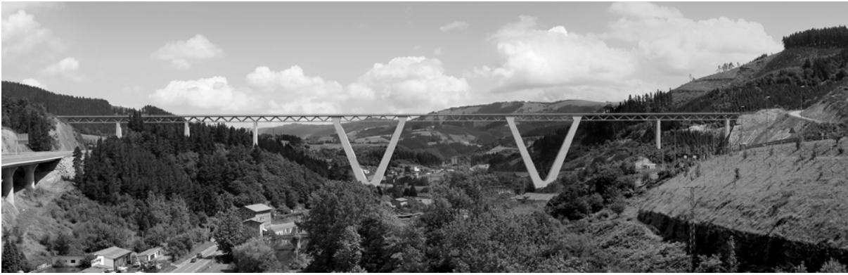
Fig. 2. View of Bergara Viaduct.
