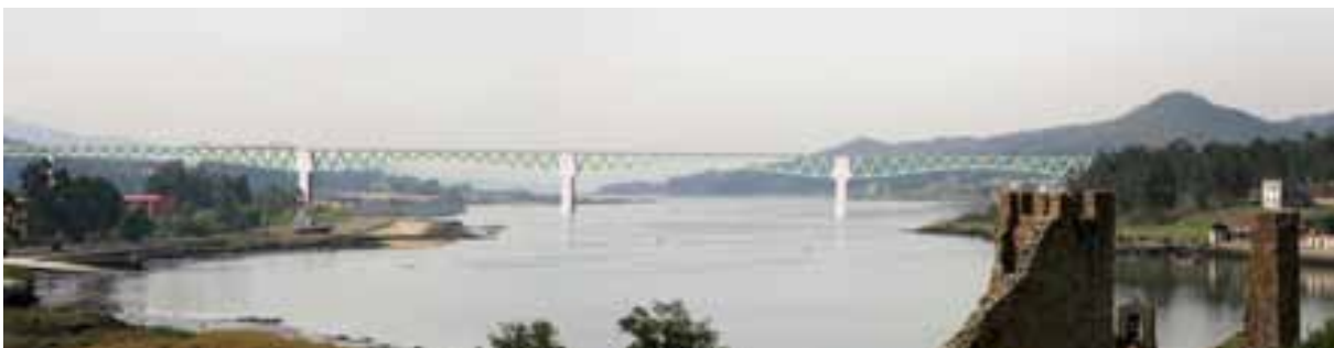
Fig. 10: View of Viaduct over river Ulla
