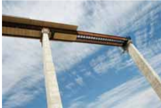
Fig. 8: Underneath view of the viaduct during
