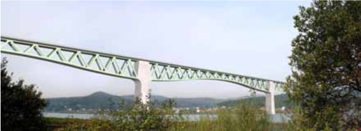
Fig. 11: Lateral view of the main span of Viaduct over river Ulla
