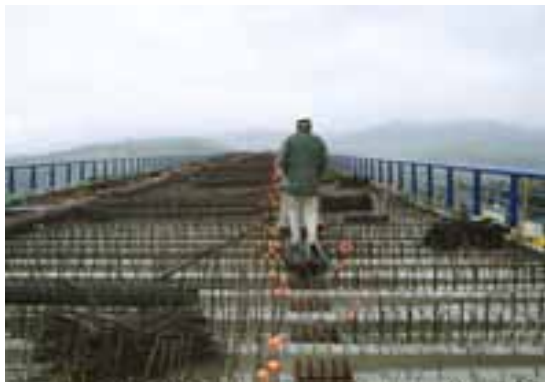
Fig. 6: View of the upper precast slabs
