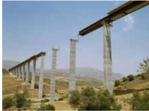
Fig. 2: View of the central piers
