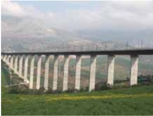
Fig. 1: View of the bridge
