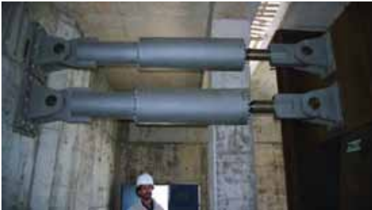
Fig. 9: Longitudinal viscous damper-shock transmission
