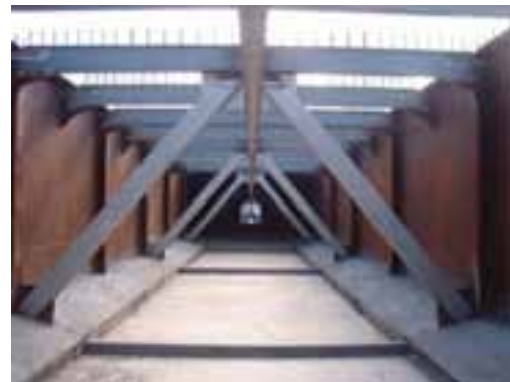
Fig. 7: View of the bottom concrete slab
