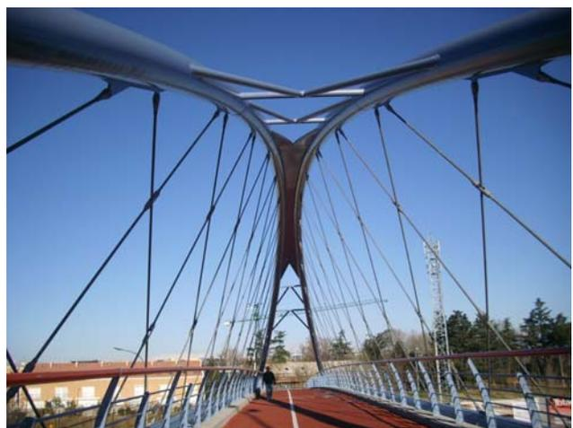
Fig.15 N-II Footbridge (80 m). Hangers detail (2007)
