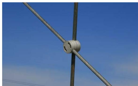
*Fig.5 Palma del Río Bridge. Hanger crossing device (2008)*
