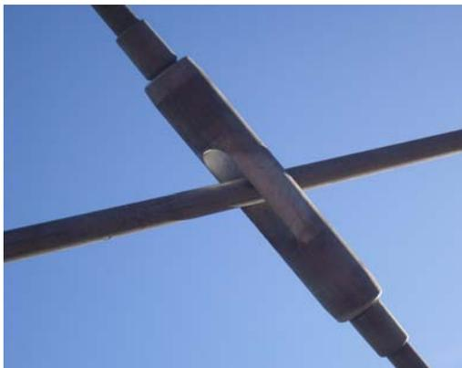
Fig.22 N-II Footbridge (80 m). Hanger crossing device
