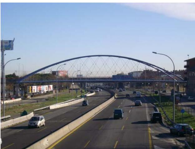
Fig.14 N-II Footbridge (network, 80 m). Front view (2007)
