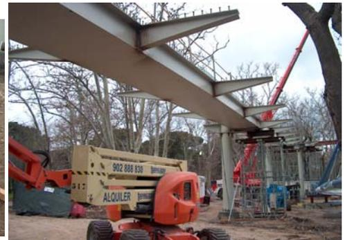
*Figs 24, 25 & 26 M-500 Footbridge (52 m) and approach viaducts. On-site metal works*
