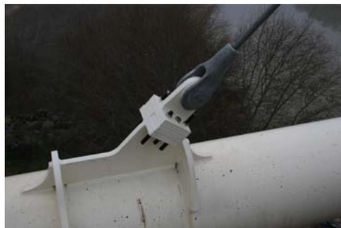
*Fig.3 Palma del Río Bridge. Hanger anchorage detail (2008)*
