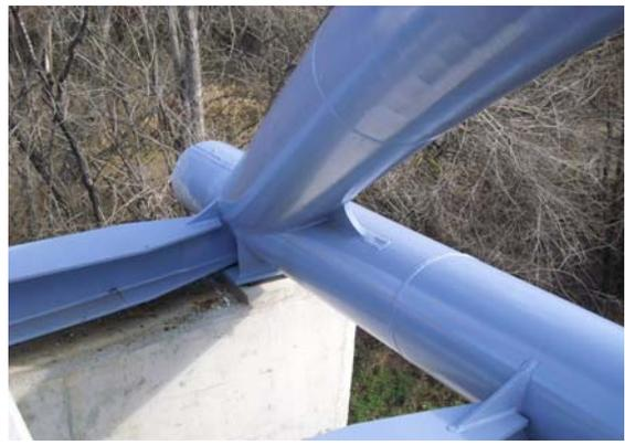
Fig.23 N-VI Footbridge (60 m). Arch-tie beam connection
