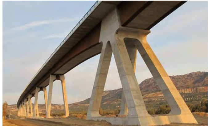
Figure 4. View of the central pier (longit. fixed point)
