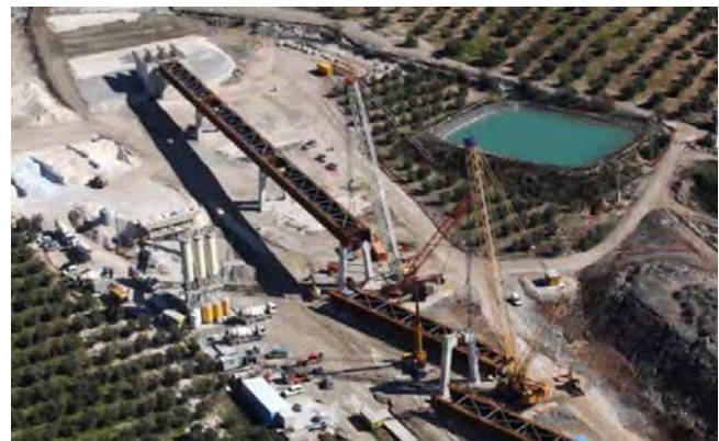
Figure 2. Deck assembly and crane erection.
