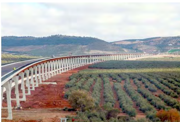
Figure 1. General view of the Archidona Viaduct.
