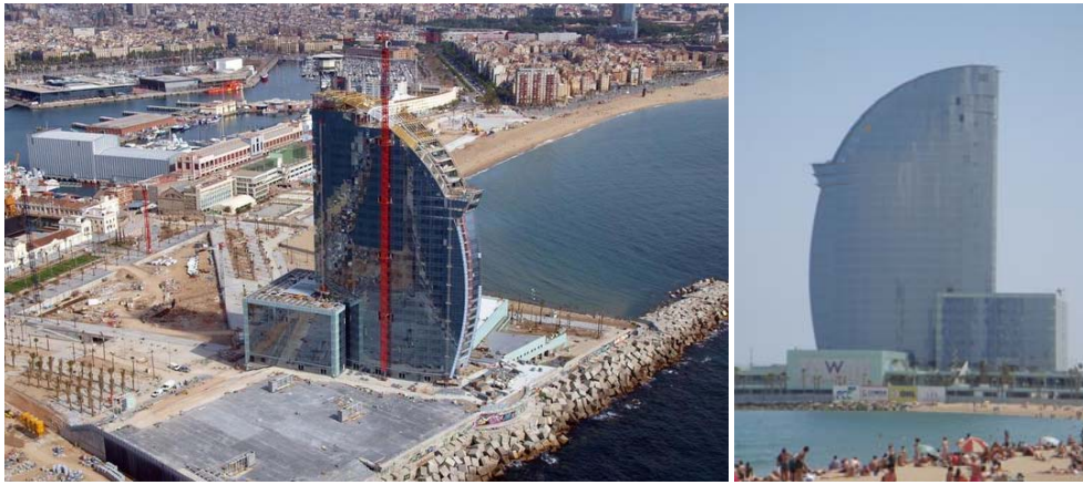
Figures 1a & 1b: Two views of the Tower and Atrium buildings.
