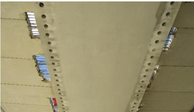
Figure 14. Bottom view of the deck with the windows in the cantilever and the holes in the bottom slab to accommodate the connection studs.
