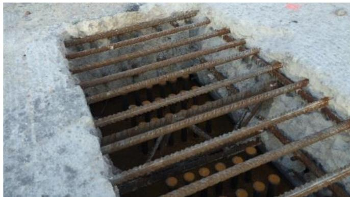
Figure 4. Hydrodemolition of a concrete slab to house stud connectors.
