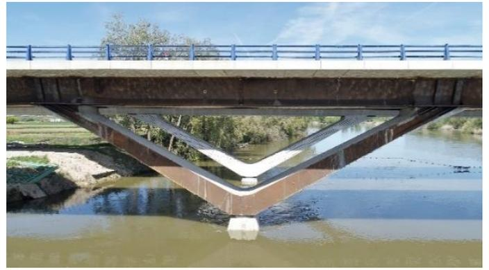
Figure 18. View of the V-shaped pier
