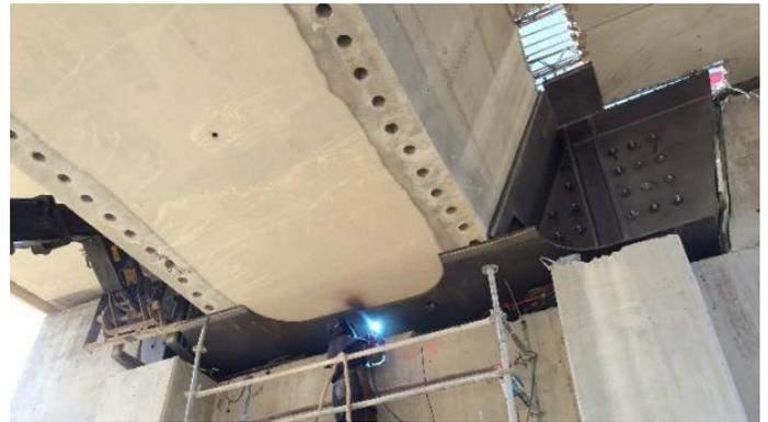
Figure 11. Welding works at abutment segments.
