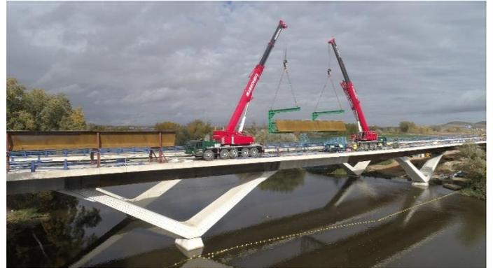
Figure 15. Erection of steel beams
