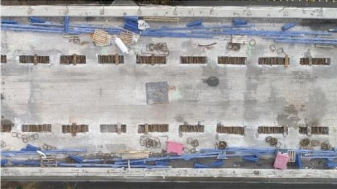
Figure 13. Plan view of the structure with the windows executed in the cantilevers to house the connecting bolts of the top flange.
