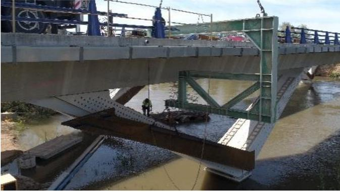
Figure 17. Steel reinforcement at V-shape piers
