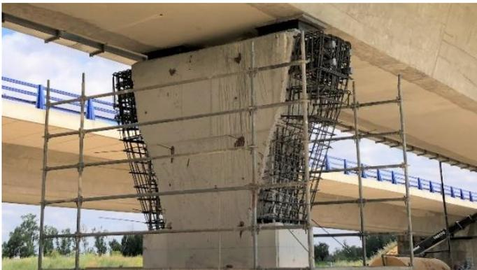
Figure 9. View of the lateral screeds in conventional piers.
