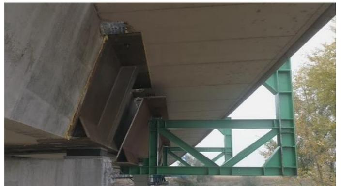
Figure 16. Erection of steel beams
